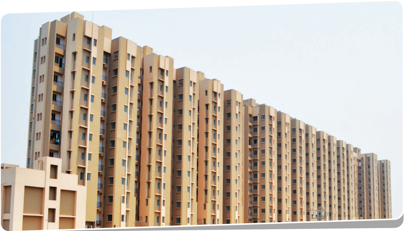
Client : Sureka Merlin Pvt. Ltd. | Total Area : 3,50,000 sqft | Location : Jajpur Road, Kalinganagar, Odisha
