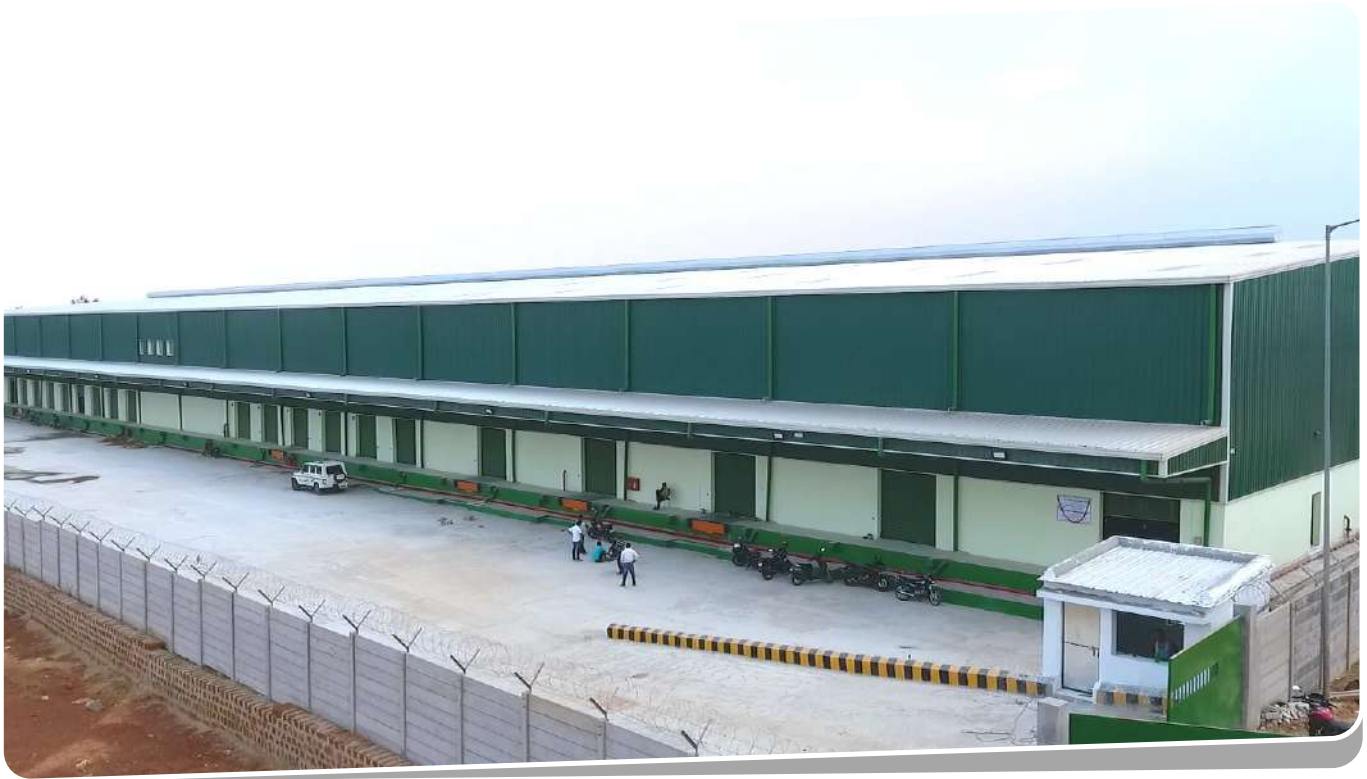
Client : Shivpujan Merchants LLP | Total Area : 1,90,000 sqft | Location : Chhatabar Industrial Area, Khordha
