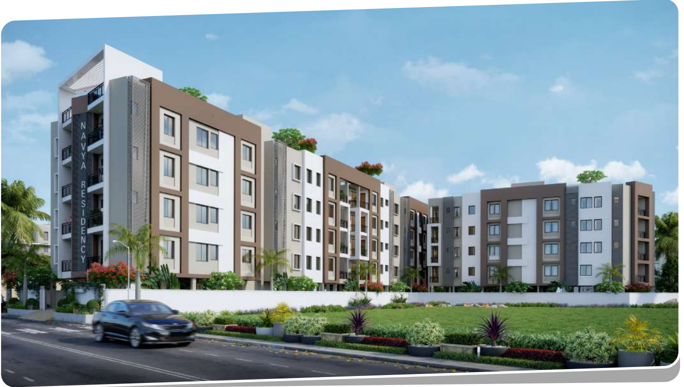
Client : Shree Ganesh Buildcon Pvt. Ltd. | Total Area : 75,000 sqft | Location : Jagnath Nagar, Mouza Pandra, Bhubaneswar
