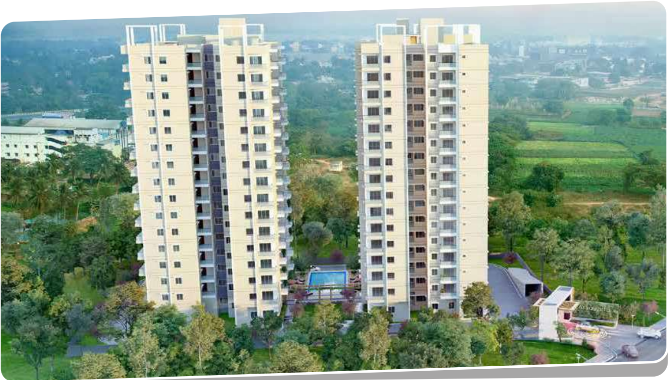
Client : Aryans Infrastructure Pvt. Ltd. | Total Area : 2,87,396 sqft | Location : Telengapentha, Cuttack, Odisha
