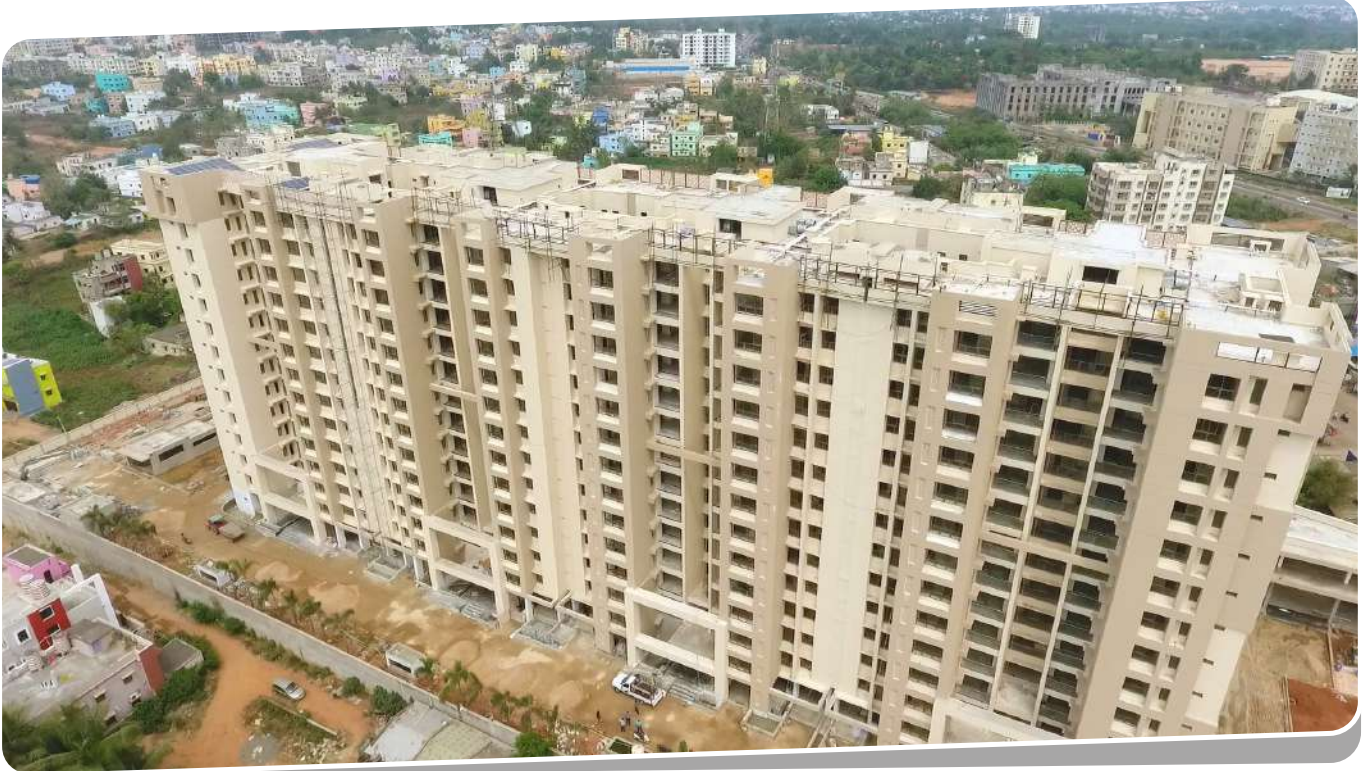
Client : Falcon Real Estate Pvt. Ltd. | Total Area : 5,30,000 sqft | Location : Sampur, Opp: Sum Hospital, Bhubanewar
