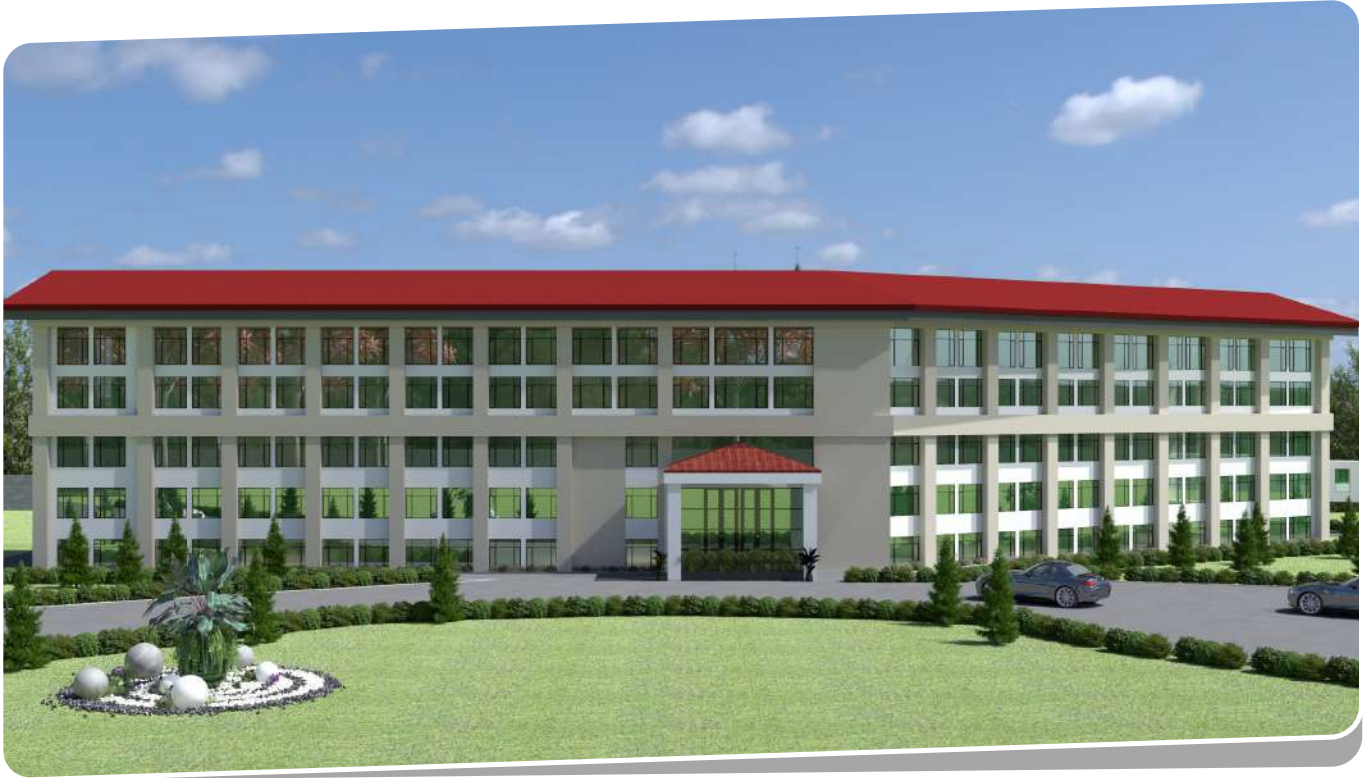
Client : HSCC (India) Limited-NEIGRIHMS | Total Area : 1,48,926 sqft | Location : Shillong, Meghalaya
