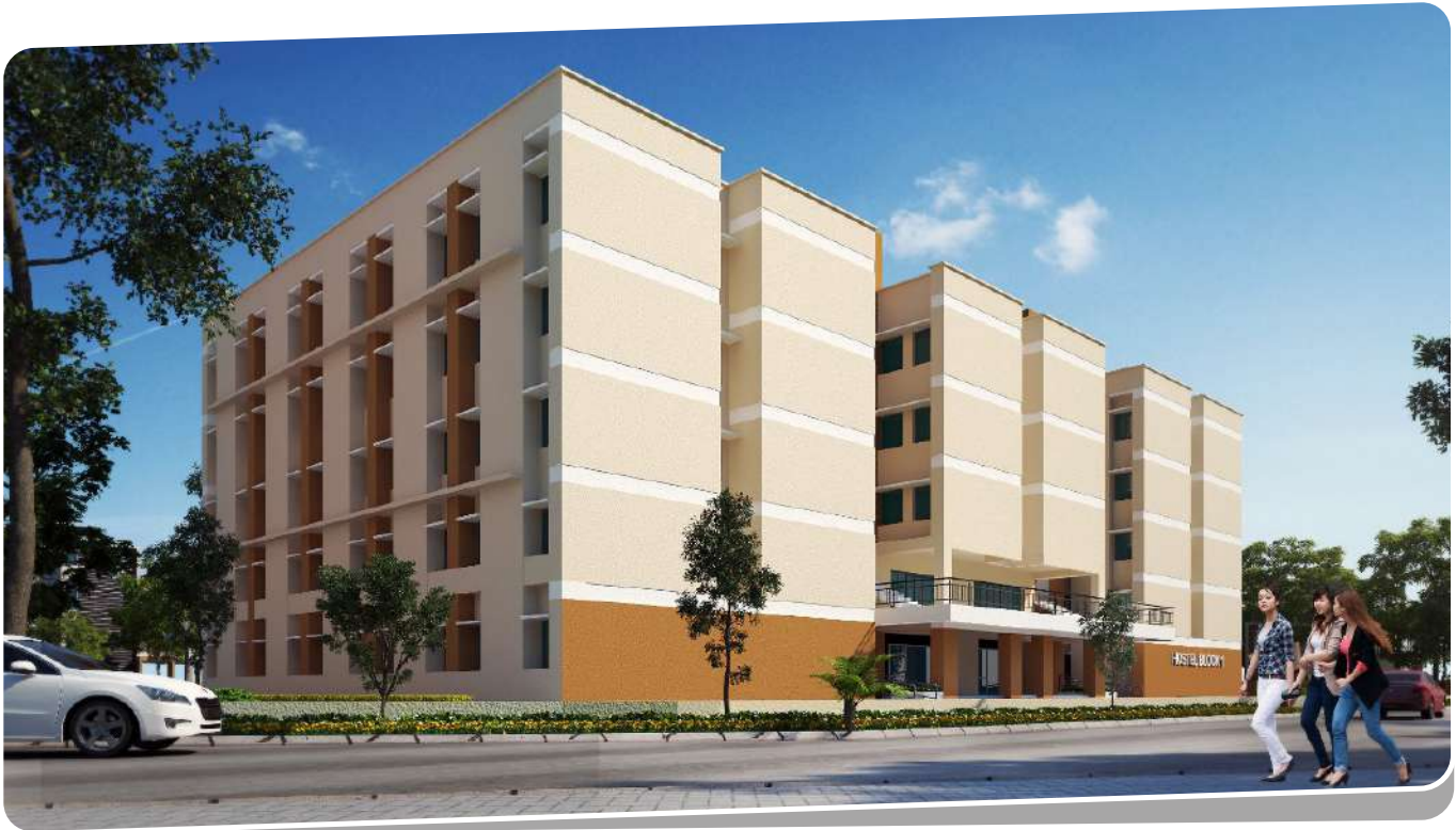
Client : Siksha O Anushandan, Bhubaneswar | Total Area : 1,25,000 sqft | Location : Campus-4, Sampur, Near SUM Hospital
