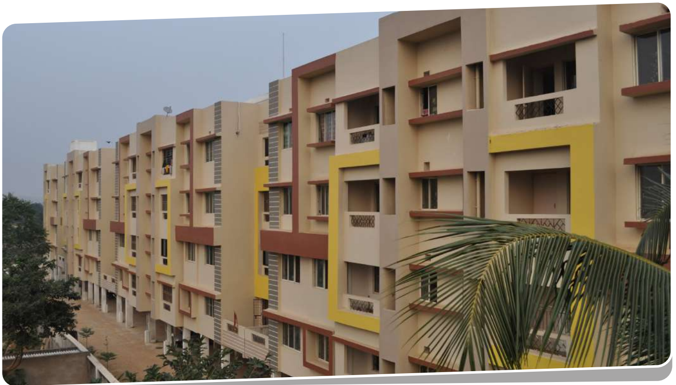
Client : Sri Jagannath Promoters and Builders | Total Area : 2,60,000 sqft | Location : Tomando, Bhubanewar
