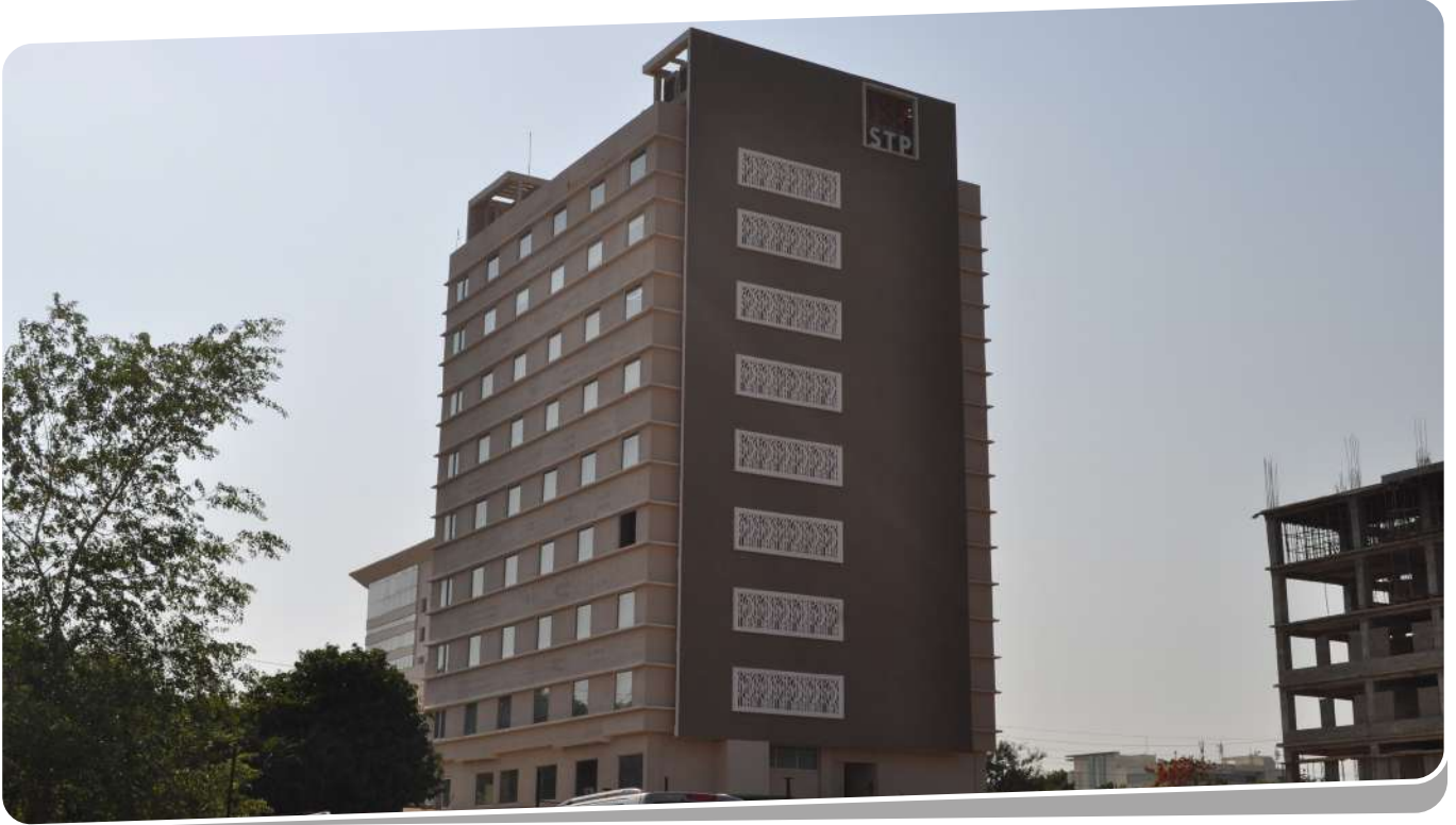
Client : JSS Consultancy Services Pvt. Ltd. | Total Area : 46,000 sqft | Location : Infocity Road, Patia, Bhubaneswar
