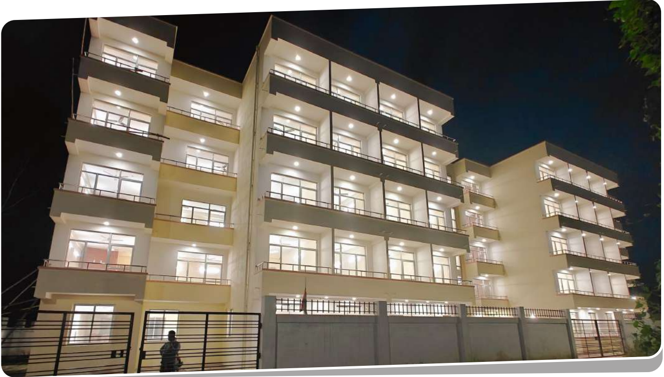
Client : Regional Institute of Medical Sciences | Total Area : 2,40,000 sqft | Location : Lamphel Road, Imphal, Manipur
