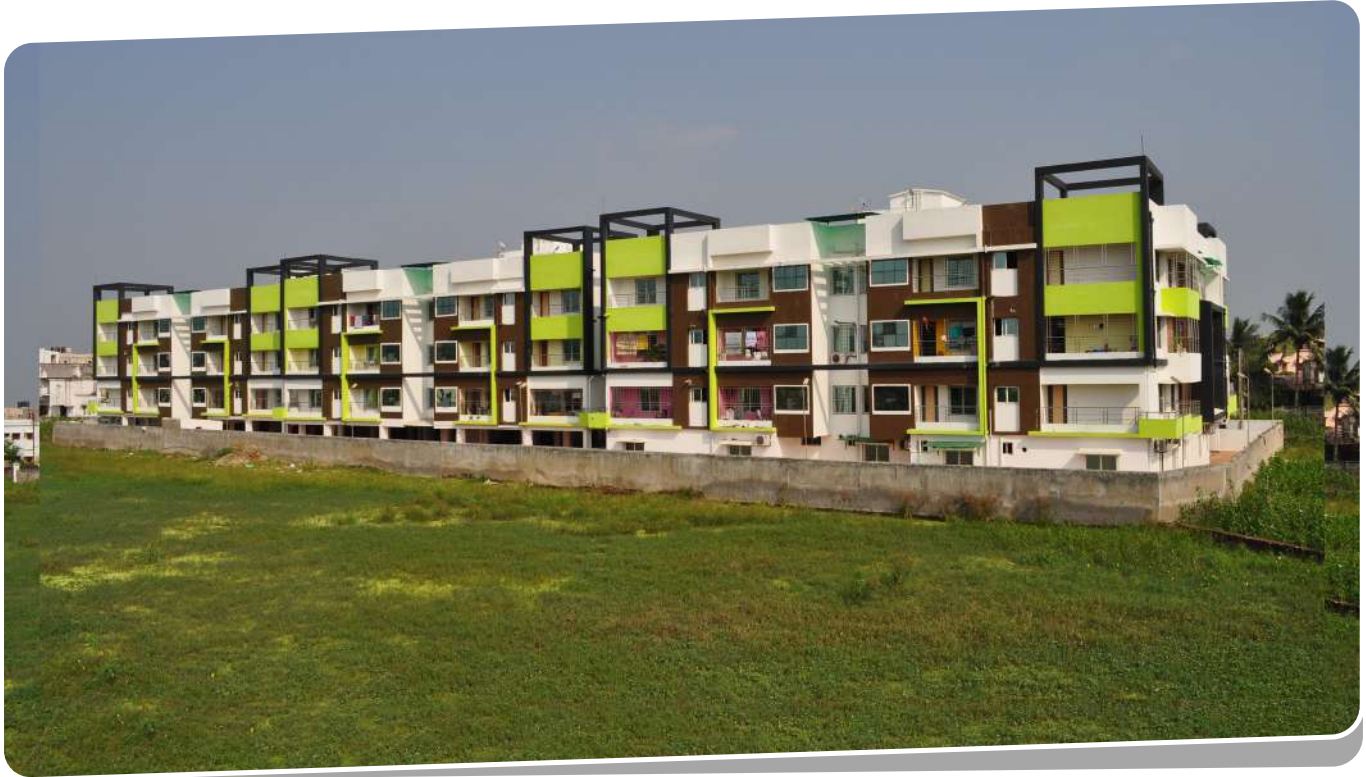
Client : PDN Developers Pvt. Ltd. | Total Area : 1,15,000 sqft | Location : ITER College, Khandagiri, Bhubaneswar
