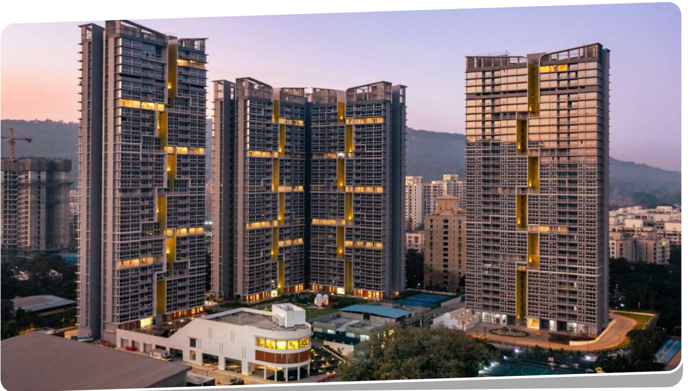
Client : Tata Realty and Infrastructure Limited | Total Area : 1,76,051 sqft | Location : Thane, Mumbai
